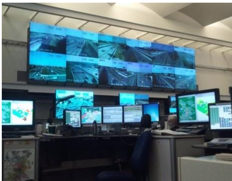
Figure 9 – Traffic management operators at CTECC use CCTV cameras, DMS and other transportation technologies to promote safety and mobility in the Region.
